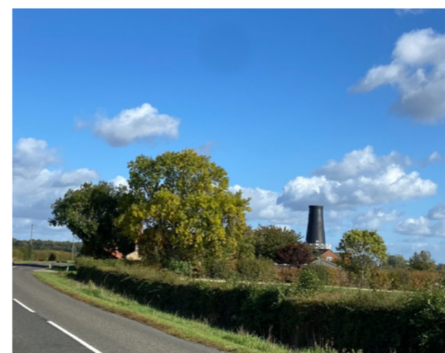
Figure 3.9: Church of St Oswald Grade II*, Blankney (top) and Scopwick Mill, Scopwick (bottom)
