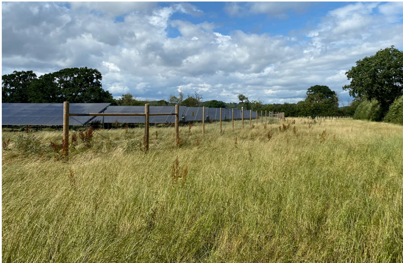
Figure 6.12: Precedent image of wooden post and wire mesh perimeter fence
